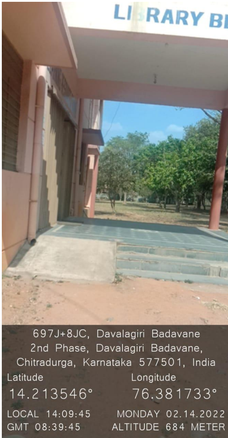
1Ramp at Library Building
